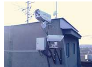
Two M1 ARTOLINK (MOSTCOM) wireless optical systems in Veseli na Morave (Czech Republic) - distances near 900 m
