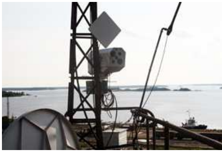
Wireless optical system M1 ARTOLINK (MOSTCOM) in Megafon company (Samara) - distance 120 m
