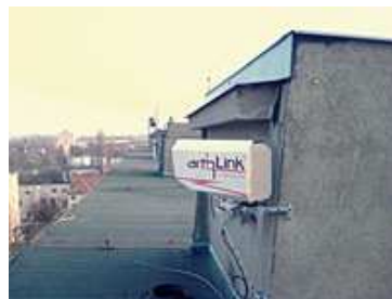
Two M1 ARTOLINK (MOSTCOM) wireless optical systems in Veseli na Morave (Czech Republic) - distances near 900 m
